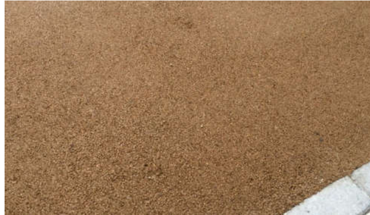
Resin Bound Gravel – Private drives
