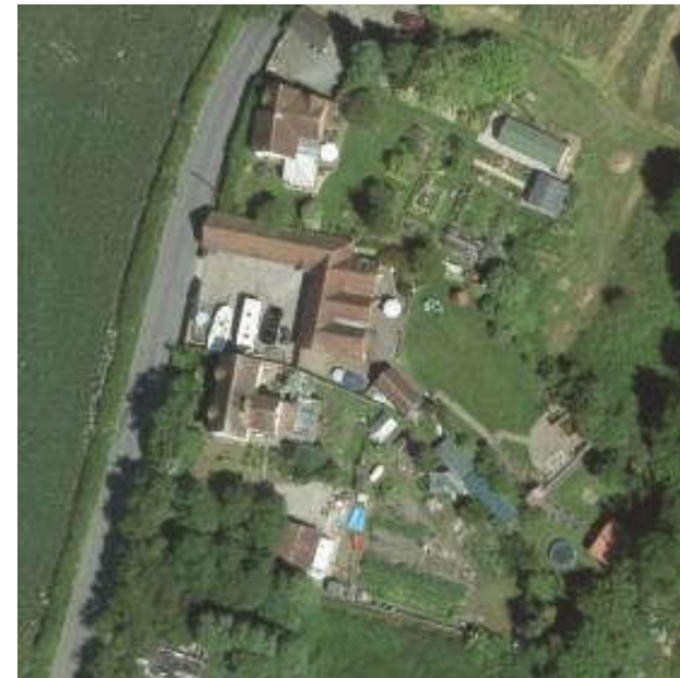
Examples of building groupings in the Arden area with interesting roof forms.
