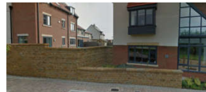
Stone wall with stone coping.
