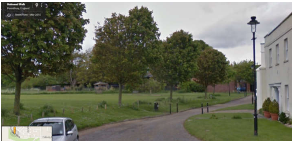
The absence of a kerb upstand allows the grass to grow over the edge of the road.
