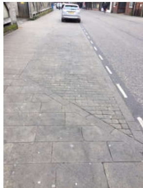
Conservation Kerbs to Parking Bays with bay laid with setts
