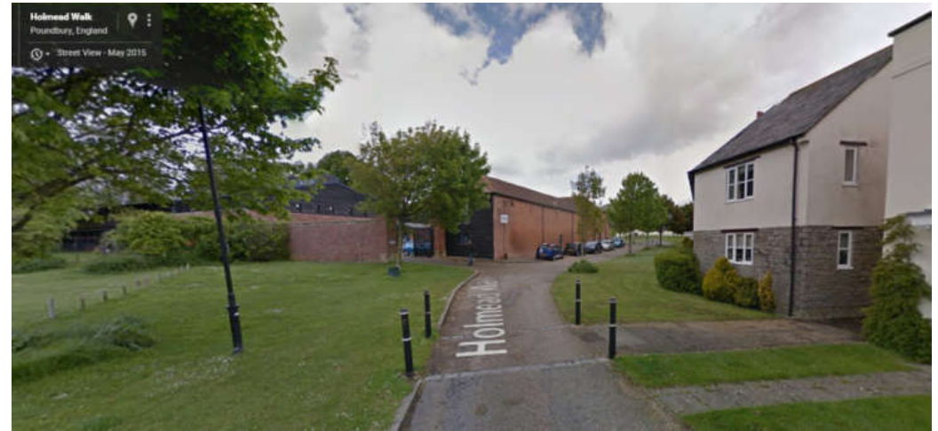
The use of bollards to narrow the carriageway at crossing points will help reduce speeds. Note the complete lack of any formal crossing points.
