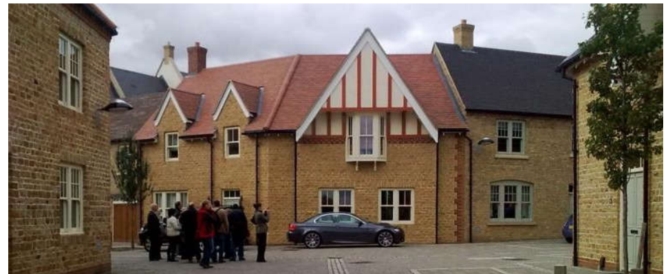
Whilst the decorative gable terminates the view down the Mews the cranked arms either side offer a deflected view telling users that the street is not necessarily a dead end.
