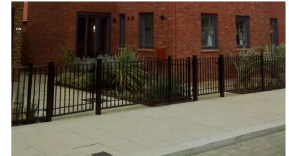
Railings to front boundary
