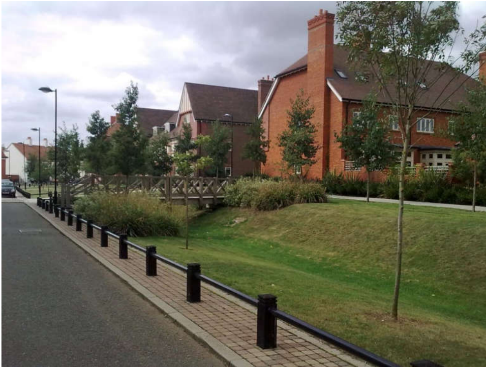
Water retention features at Upton, Northampton have been positively integrated into the design
