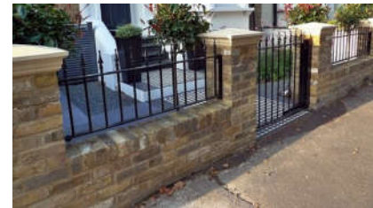
Masonry wall topped with railings.
