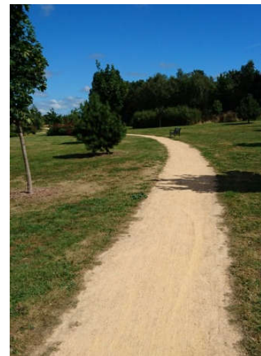
Unbound Quality Gravel – foot path/cycle paths through open space and open countryside
