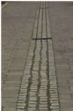
Granite Cobble drainage channel
