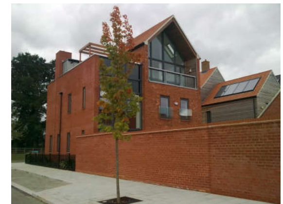
Brick wall with brick and tile coping.
