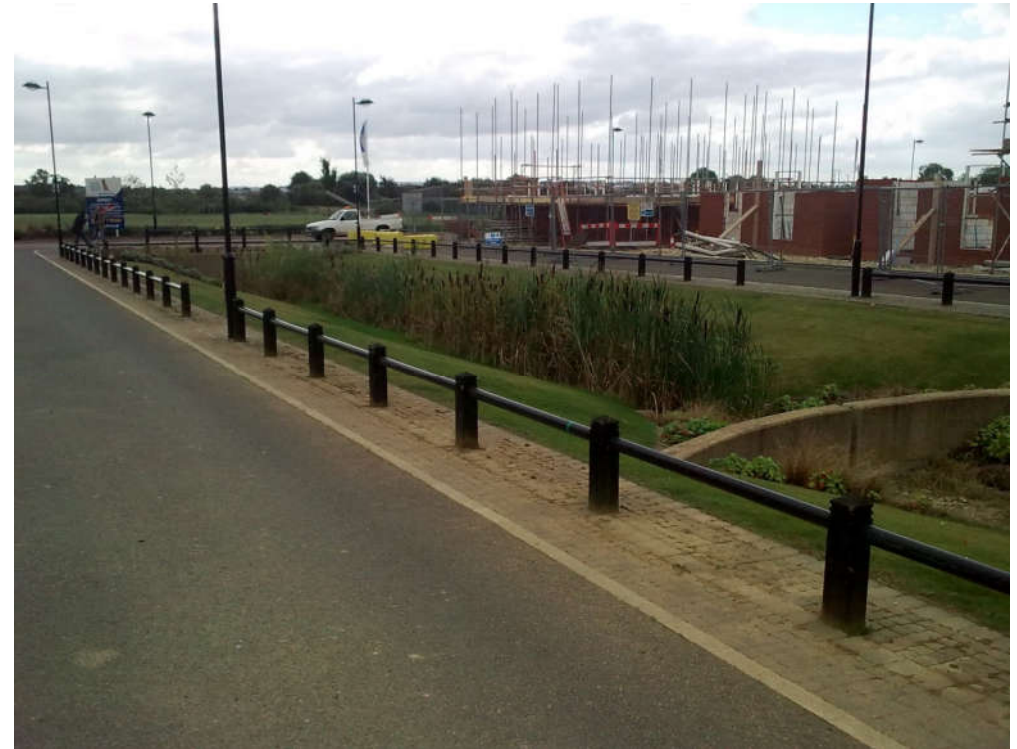
Grey to Green, Sheffield (left) and reed beds, Upton (above). Swales are used to retain rainwater and clean it of its pollutants via the stone, underlying soils and planting.
