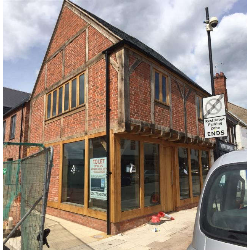
New build timber frame building. Designed and constructed to a very high standard. This demonstrates that a traditional building technique such as this can be recreated if done properly. Given that this style of building is prevalent in the Arden it should not be dismissed off hand but caveated that any proposal for this form would need to be to this standard.
