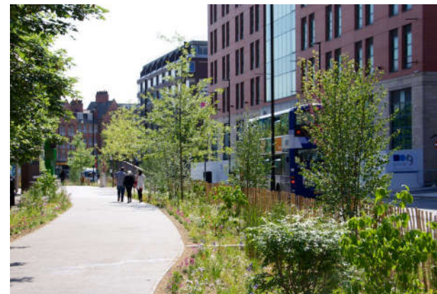
Grey to Green, Sheffield (left) and reed beds, Upton (above). Swales are used to retain rainwater and clean it of its pollutants via the stone, underlying soils and planting.
